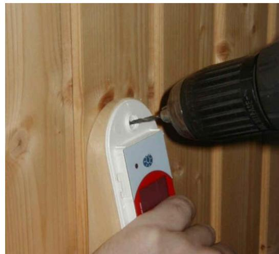
3. Then fix the controller using a screw to the wooden base. Once you have ensured that the controller is straight as regards the base, drill through the lower plank and screw the controller also as regards its lower part.
