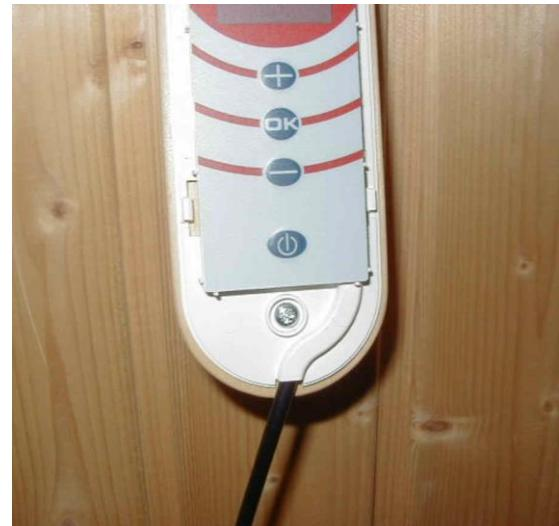
5. Locate the controller frame into its place. The frame is located in its place by pressing with the hands. Remove, using for example a knife, the pre-worked plastic part reserved for the cable.
